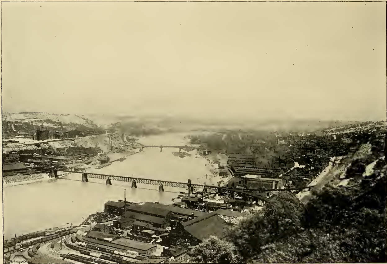
View of South Side and Panhandle R. R. Bridge.
